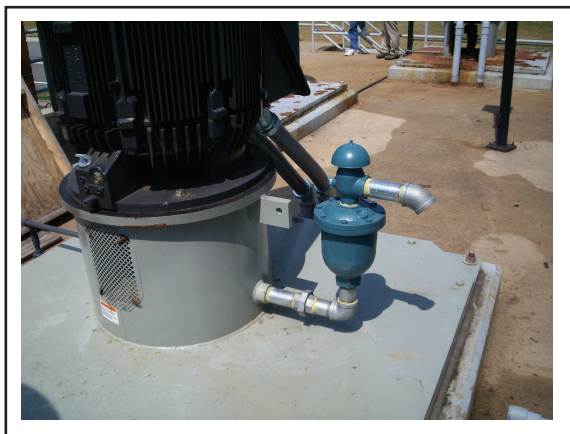
Air/Vacuum Valve with Dual Port Throttling Device
