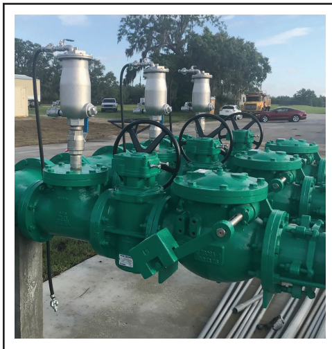
Single Body Wastewater Combination Air Valve
