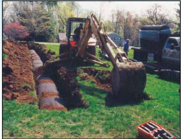
Trench installation demonstrating minimal disturbance of land.
