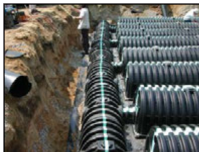
External manifold using CULTEC HVLV® 180 Header System
