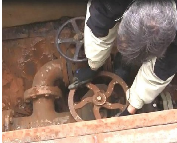
Figure 13 – Inlet Valve
