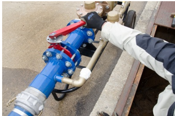
Figure 6 – Release Trapped Air– High Side
