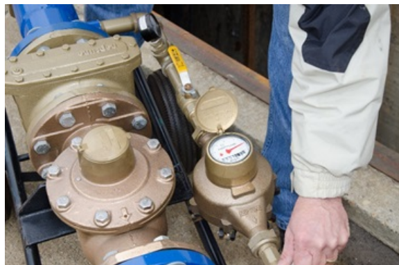
Figure 7 – Release Trapped Air – Low Side
