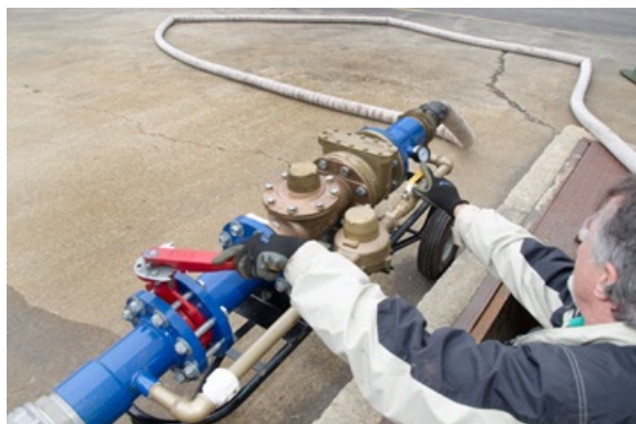
Figure 18 – High Side Valve on Reference Meter
