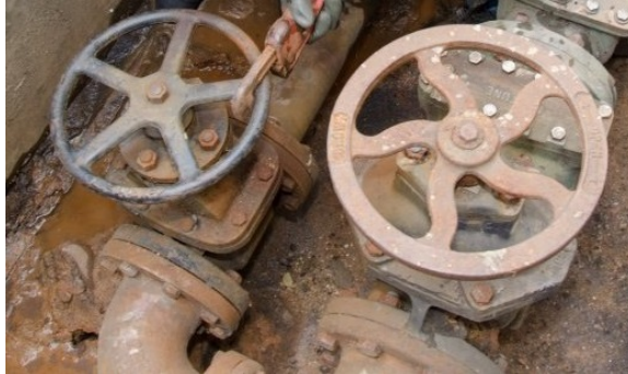
Figure 20 – Bypass Valve
