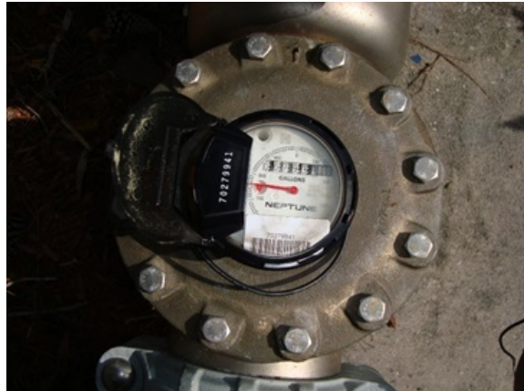
Figure 8 – Register – High Side
