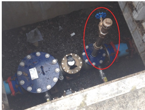
Figure 2 – HP PROTECTUS® III Test Port
