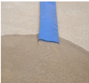
Figure 27 Clear Water After Back-flush
