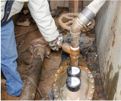
Figure 28 Test Riser Valve Attached to Meter Under Test
