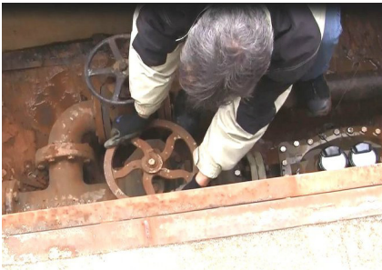
Figure 24 Inlet Valve
