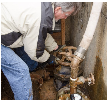
Figure 13 Shutting the Outlet Valve
