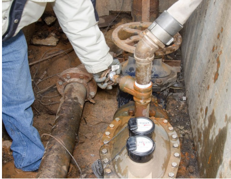
Figure 11 Opening the Test Riser Valve
