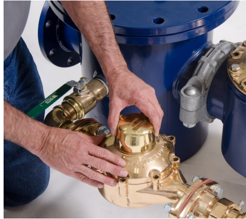
Figure 10 – Removing the Register
