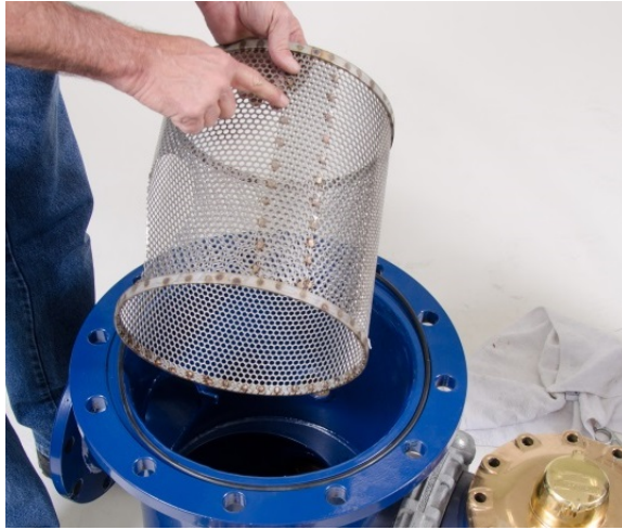
Figure 32 – Inspecting the Basket
