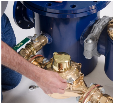
Figure 9 – Removing the T-10 ® Bolts
