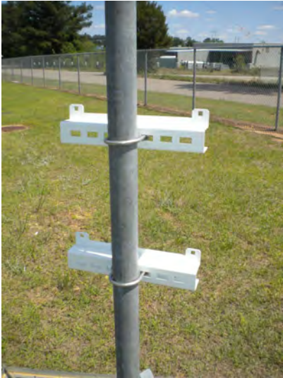
Figure 34 – Installing Pole Brackets
