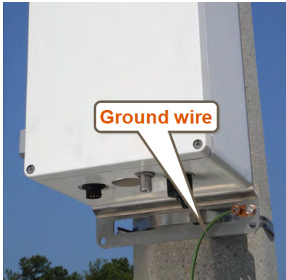
Figure 63 – Attach Ground Wire
