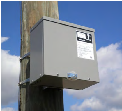
Figure 67 – UPS Attached to a Large Pole
