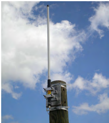
Figure 53 – RF Antenna Bracket
