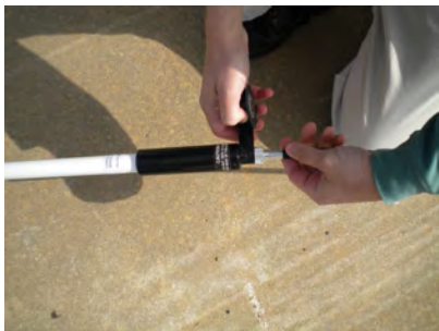
Figure 83 – Weatherizing RF Antenna
