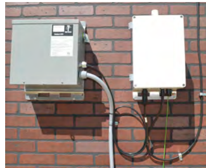
Figure 2 – AC-Powered Wall Unit
