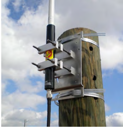
Figure 54 – Coax Cable Attached
