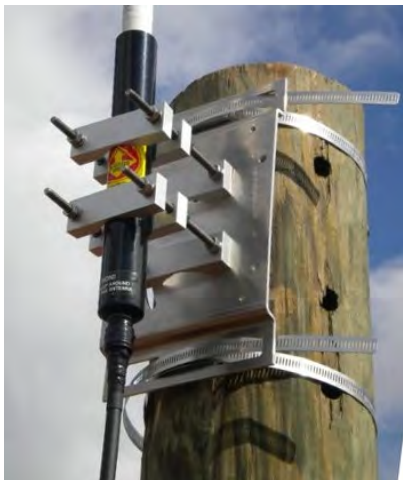
Figure 55 – Weatherized Connection
