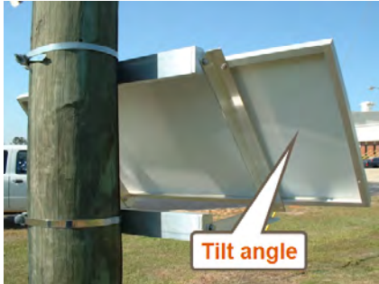
Figure 61 – Mounted Solar Panel
