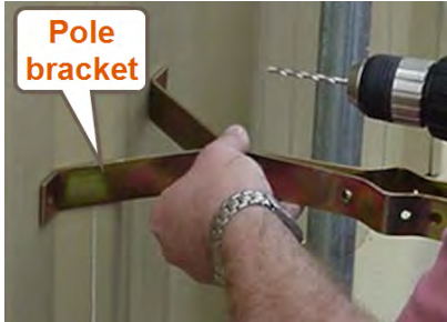
Figure 79 – Securing Pole Bracket
