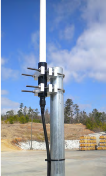
Figure 84 – RF Antenna to Mast
