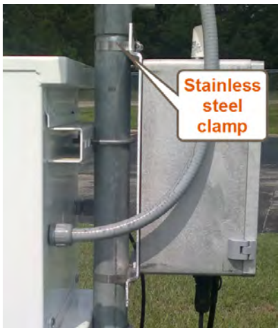
Figure 41 – Positioning the Gateway
