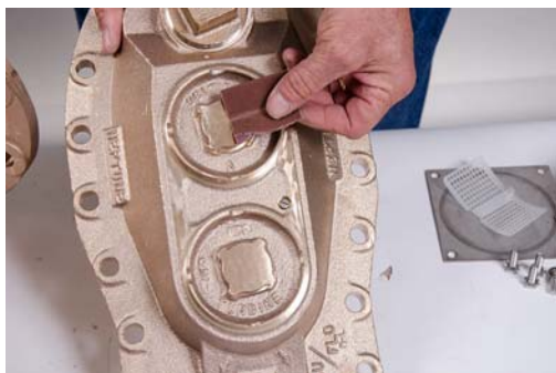
Figure 22 Cleaning Under the Registers
